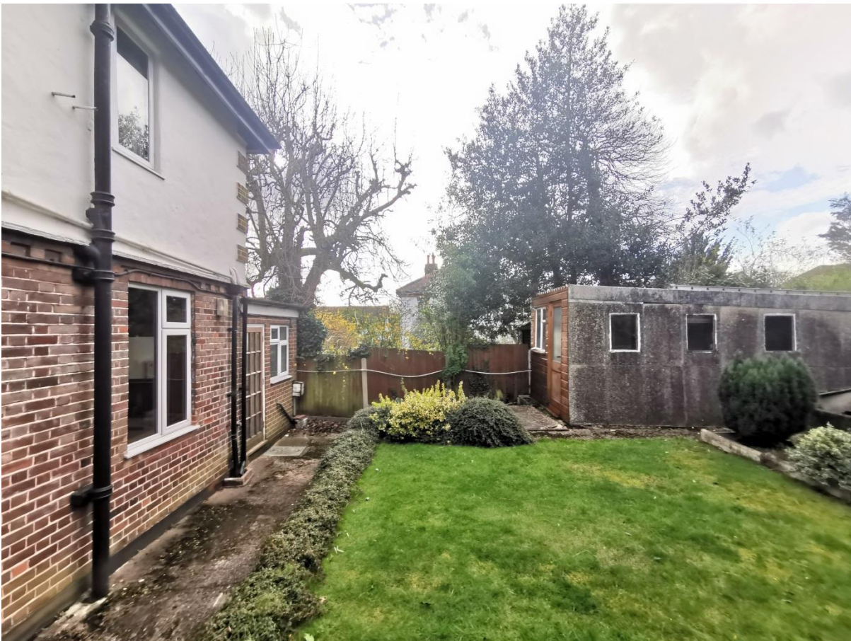
Figure 3 Rear elevation facing towards Nower Hill
