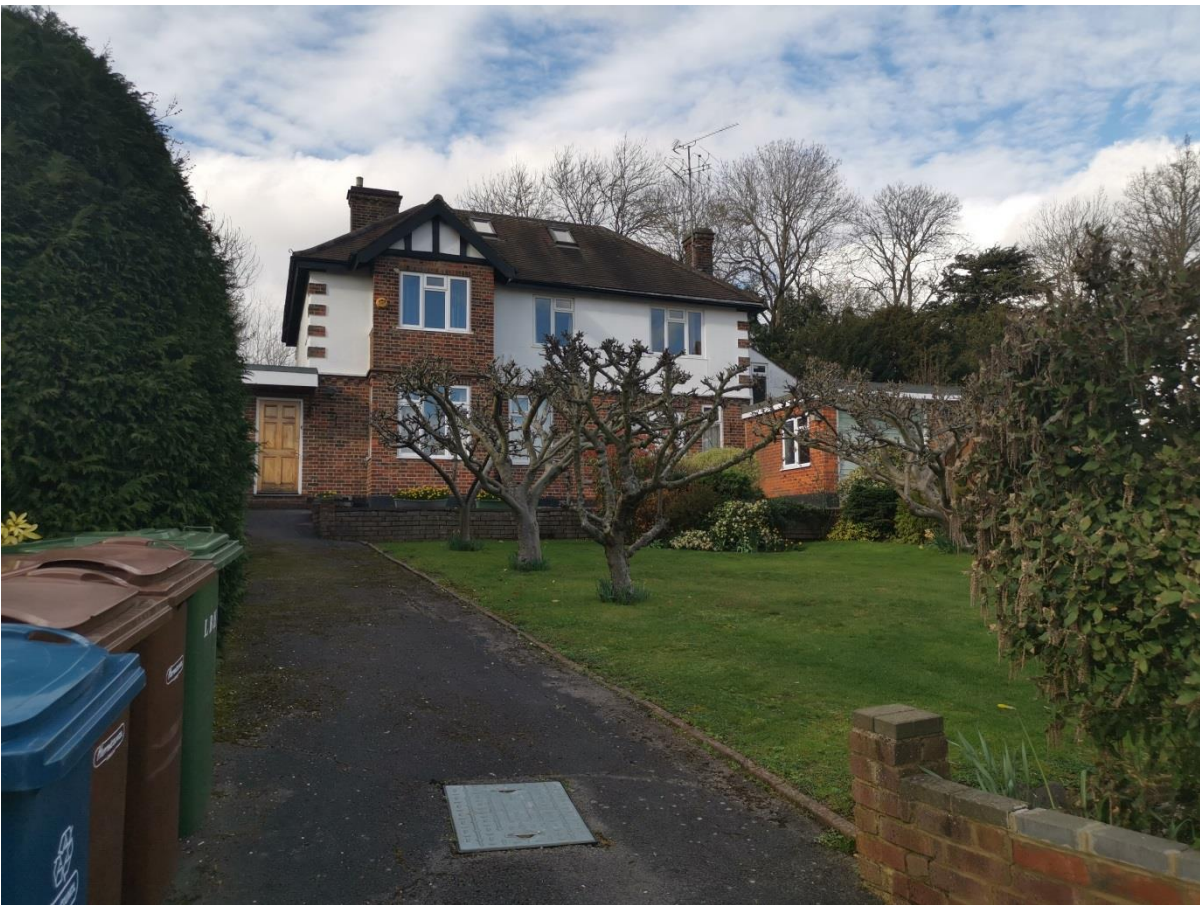
Figure 1 View of property looking north from Mayfield Drive
